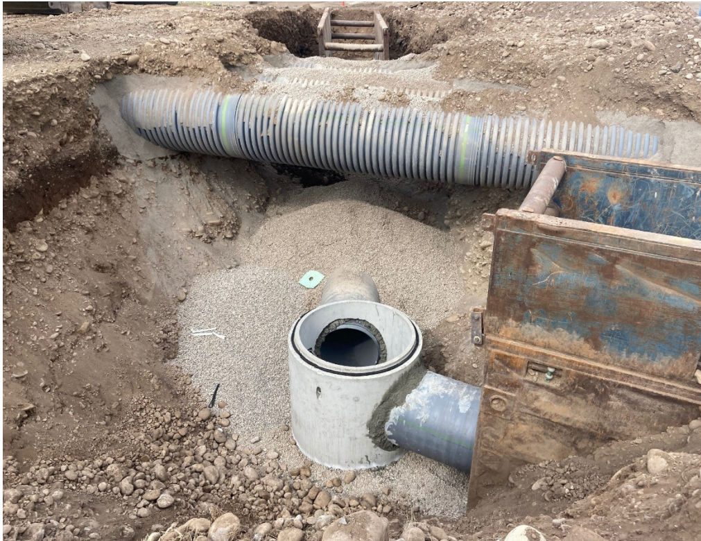
Storm Drainage System Installation
