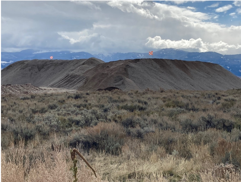
Base Course Aggregate Stockpile (Screened and Crushed from Native onsite Materials)
