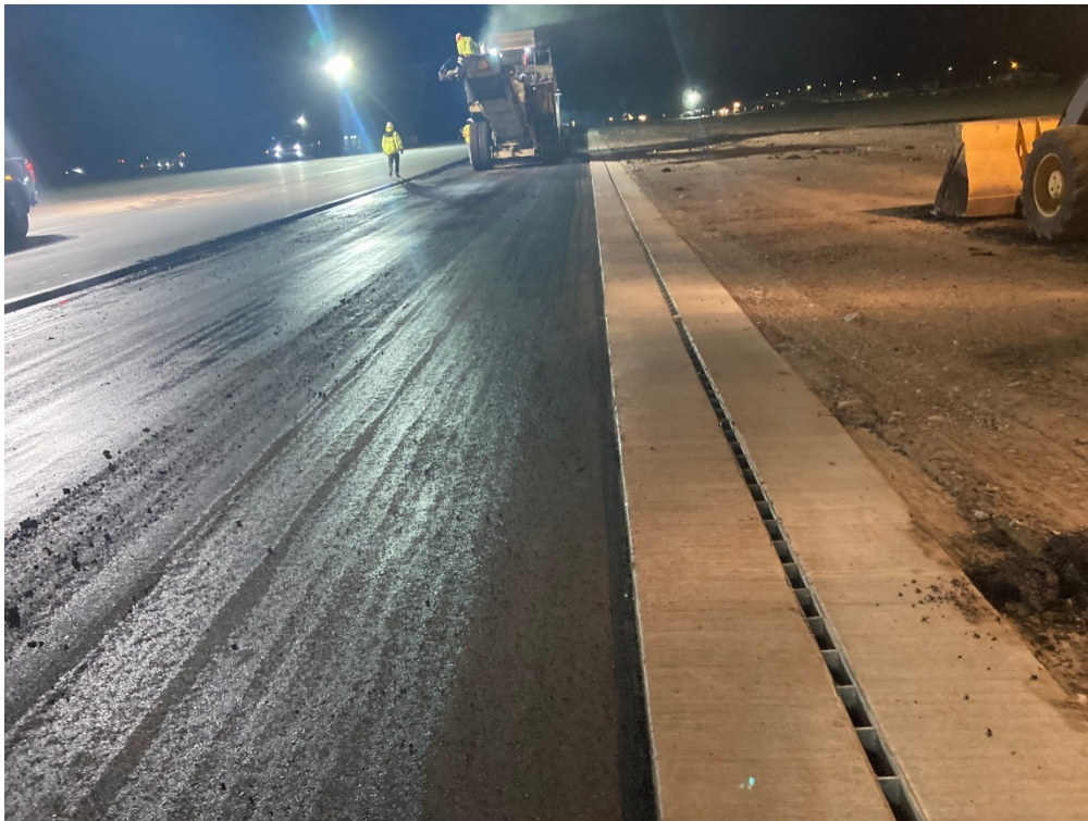
New Surface Runoff Capture System (Perimeter Slot Drains)
