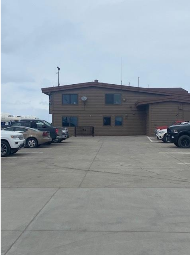
Location of proposed Airport administration building and Airport Fire House in background.
