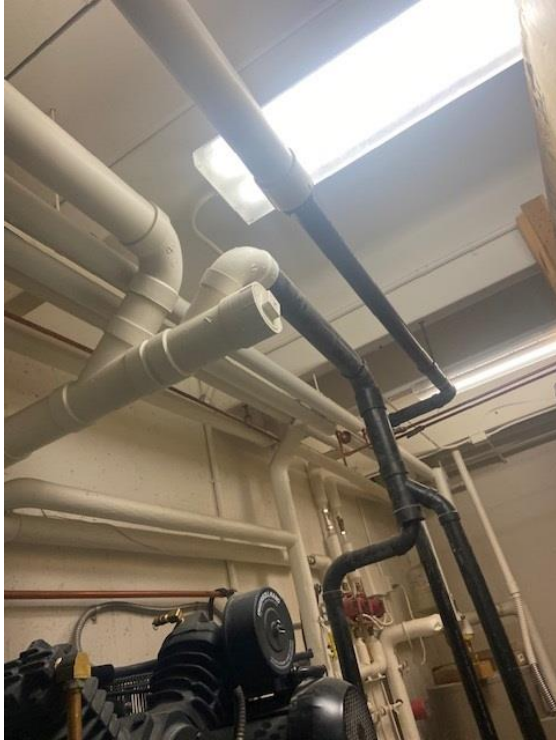
Plumbing utility tie in location.
